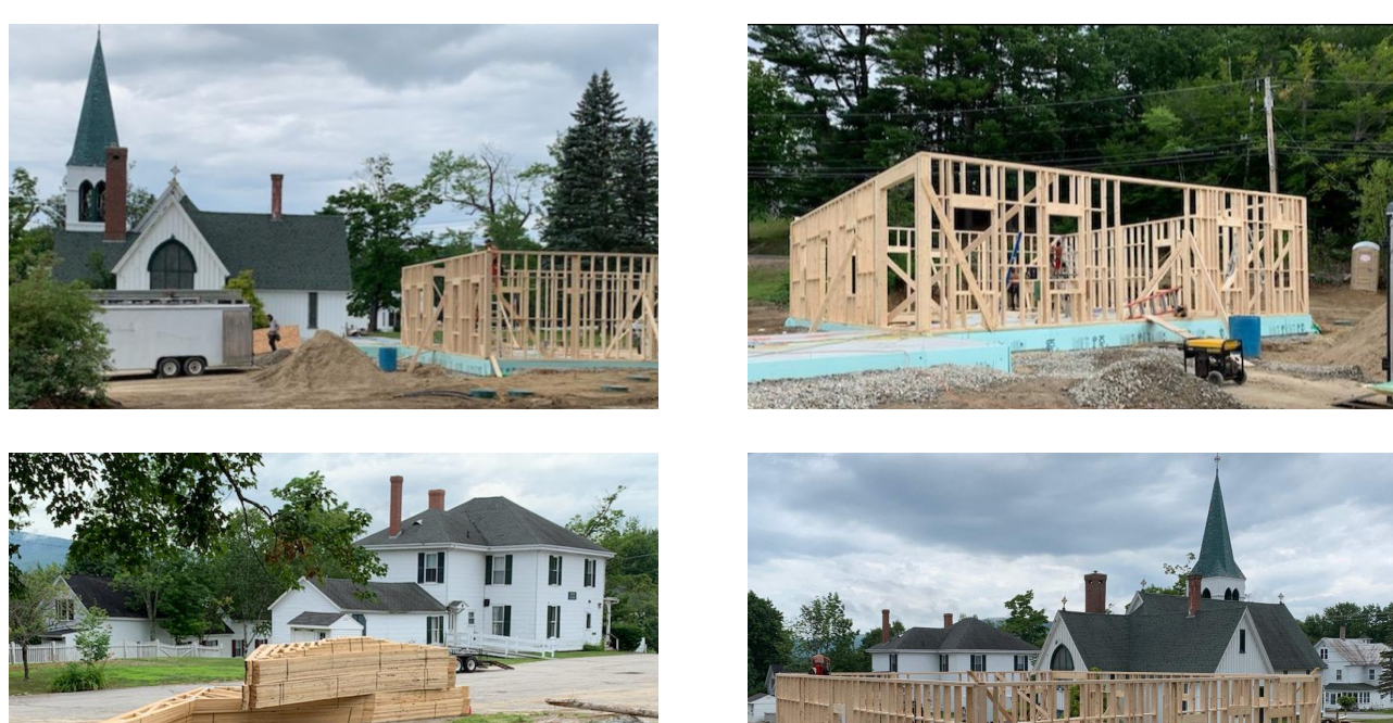
Framing, trusses on site -- lots of visible progress!
